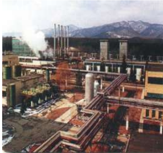
The Feldioara Uranium Ore Processing Plant
